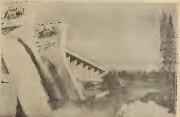
This is a hydro-electric dam near Onkari, at the top of the Gulf of Bothnia, in Northern Finland. Developments such as this are symbols of Finland's growing industrial importance since the war, reported Toronto students after their Hart House-sponsored work tour of Finland. Most of the students were from the professional faculties of the University. They worked in divergent locations, ranging from a metallurgical laboratory to a hotel, and from the south of Finland to north of the Arctic Circle.
